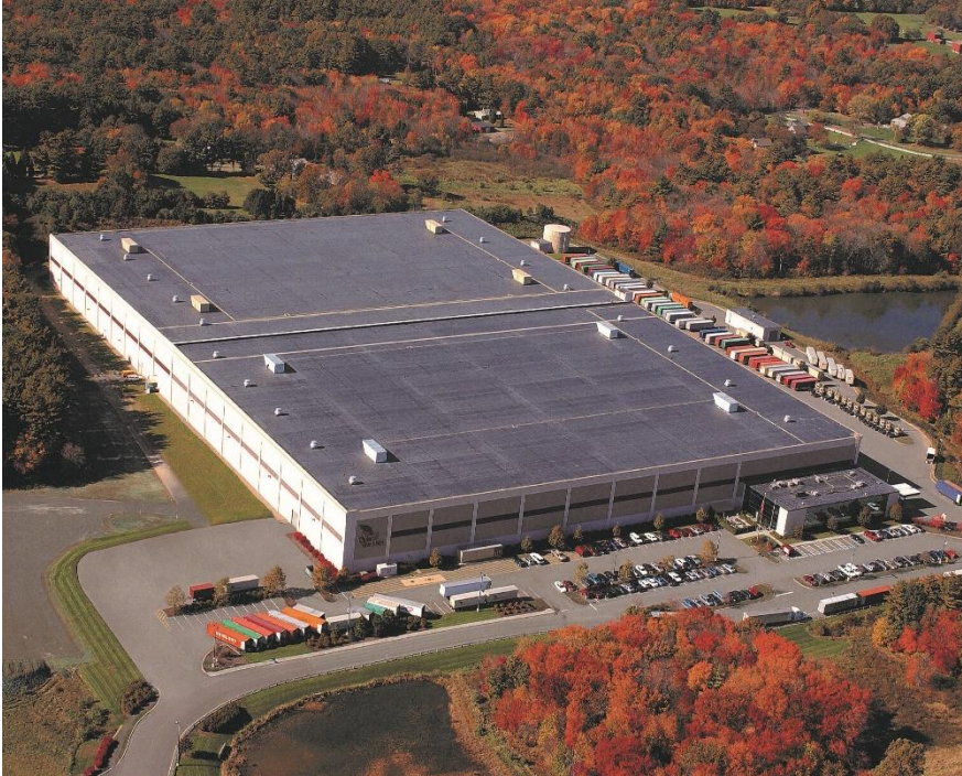
Singly ply, reinforced EPDM membrane mechanically fastened and representative of 60 and 75 mil thicknesses
